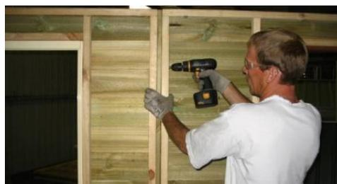
5. Continue positioning and attaching the remaining walls as per steps 3 and 4 above.
