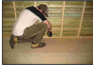
7. Place a gable top onto the wall. Centre the gable top on the wall, ensuring it finishes flush with the wall on either end. The cladding overhang on the gable top should be pulled firmly against the gable wall cladding. Fix into position using three 70mm bugle screws placed approximately 400mm from each end, and one in the centre. Screw up through the top plate of the wall into the bottom plate of the gable top. Follow the same process to fit the gable top to the other gable wall.
