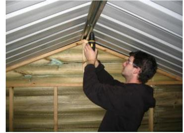
11. Shed roof facias come as two matched pairs, each containing a left and a right hand fascia board. Position the facias ensuring the top edge of the fascia is flush with the top of the roof panel, with one end central against the ridge beam. Screw through the fascia into the channel frame of the roof using three 40mm wing tip screws, one toward each end and one in the centre.
