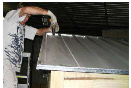
10. Secure the roof into the beam from inside the shed using 20mm tech screws at equal spacings along the beam length, screwing through the beam and into the channel frame of the roof panel.
