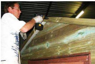
12. Once shed is erected and square, put the door into position, line the hinge holes up with the pilot holes in the jamb and screw.
