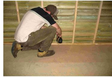
7. Place a gable top onto the wall. Centre the gable top on the wall, ensuring it finishes flush with the wall on either end. The cladding overhang on the gable top should be pulled firmly against the gable wall cladding. Fix into position using two 70mm bugle screws placed approximately 400mm from each end. Screw up through the top plate of the wall into the bottom plate of the gable top. Follow the same process to fit the gable top to the other gable wall.
