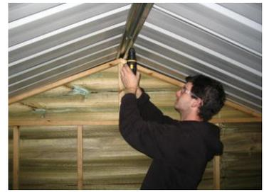
12. Screw through each corner of the top plate on the truss into the ridge beams using four 20mm hex screws.
