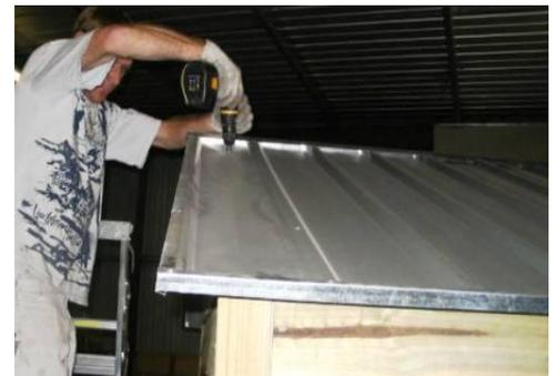
10. Repeat steps 8 and 9 to fit the other half of the roof. The second roof sections should overlap the end ribs of the sheets on the first roof sections. The protruding flap of the capping on one ridge beam should pass under the flush finished capping on the other.
