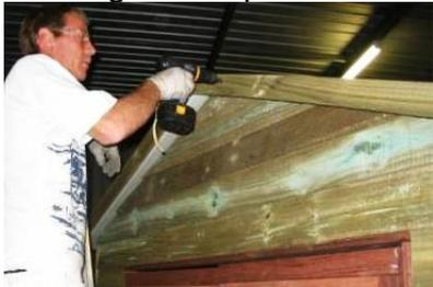
12. Once the shed is erected and square, put the door into position. Line the hinge holes up with the pilot holes in the jamb and screw.
