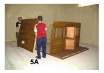
7. After ensuring the bottom of the front wall is still firmly positioned hard against the particleboard, fix the walls to the using three 70mm bugle screws through the bottom plate of wall into the flooring joists – one toward each end and one in middle.
