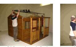
Position one 595mm length facia on the end of the veranda roof aligned with the front veranda facia. Screw through the facia the channel frame of the roof using one 40mm wing tip screw each end. Repeat this process to fix the second facia on the other end of the veranda.
