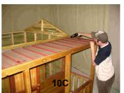
11. Position the 2670mm long roof facia onto the edge of the roof panel, flush to the top and overhanging 20mm on each end. Secure into position using four 40mm wing tip screws driven through the facia and into the channel frame of the roof panel, screw above each balustrade post. Secure the facia to the balustrade posts using four 50mm particleboard screws driven through the facia into the posts.
