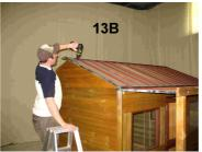
Position one 595mm length facia on the end of the veranda roof aligned with the front veranda facia. Screw through the facia the channel frame of the roof using one 40mm wing tip screw each end. Repeat this process to fix the second facia on the other end of the veranda.
