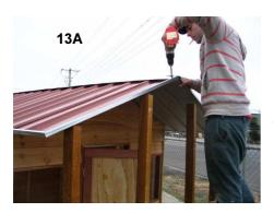
13. Using four 20mm tech screws, screw through the edge corners of the flashing on the ridge beam into the roof panel channel.
