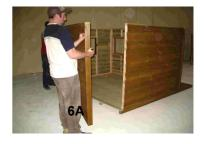
7. After ensuring the bottom of the front wall is still firmly positioned hard against the particleboard, fix the walls to the using two 70mm bugle screws through the bottom plate of wall into the flooring joists.
