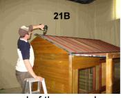
Position one 605mm length facia on the end of the veranda roof aligned with the front veranda facia. Screw through the facia the channel frame of the roof using one 40mm wing tip screw each end. Repeat this process to fix the second facia on the other end of the veranda.
