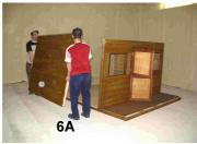
7. After ensuring the bottom of the front wall is still firmly positioned hard against the particleboard, fix the walls to the using two 70mm bugle screws through the bottom plate of wall into the flooring joists.
