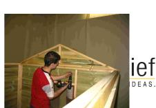
ensuring it finishes flush with the wall on either end. The cladding overhang on the gable top should be pulled firmly against the side wall cladding. Fix into position using two 70mm bugle screws placed approximately 400mm from each end. Screw up through the top plate of the wall into the bottom plate of the gable top.
