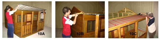
11. Position the 2115mm long roof facia onto the edge of the roof panel, finishing 25mm above the top and overhanging 20mm on each end. Secure into position using four 40mm wing tip screws driven through the facia and into the channel frame of the roof panel, one screw above each balustrade post. Secure the facia the balustrade posts using four 50mm particleboard screws driven through the facia into the posts.
