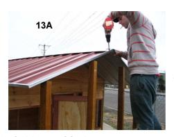
20. Using four 20mm tech screws, screw through the edge corners of the flashing on the ridge beam into the roof panel channel.
