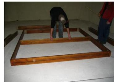
2. Check the frame is square by measuring the diagonals – both should be equal. If not move a corner as required to achieve square.
