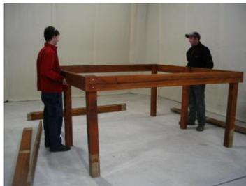
7. Use a level on top of the bearers and on the sides of each post as you work from post to post. Screw through the centre of the bearer into each post.
